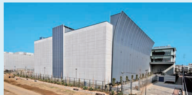
Mitaka Data Center EAST exterior
