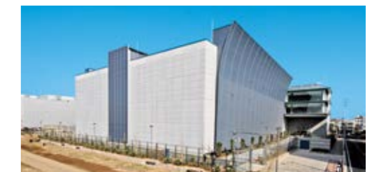
Mitaka Data Center EAST exterior
